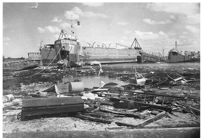
View of typical damage in Buckner Bay.
